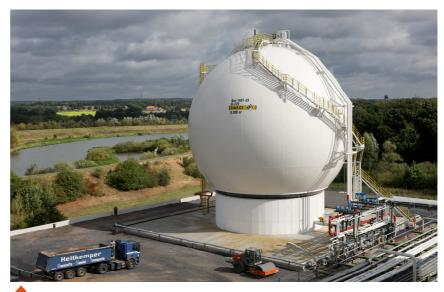
Segments welded together to form a complete sphere. Fit and quality is an absolute requirement. The Deform sphere in above is nearly 26 meters in diameter!
